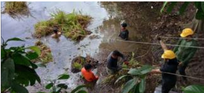
Figure 57: Rope hauling systems being readied to pull out the netted Grass Sudds
